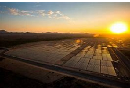
Arlington Valley Photovoltaic Solar Panels
