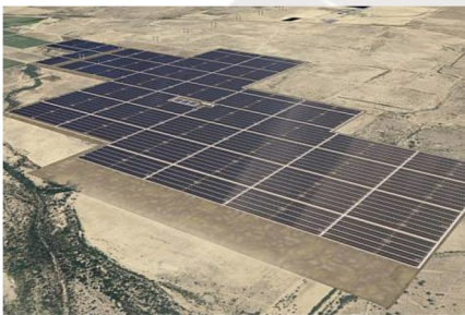
Aerial View of Arlington Valley Solar Energy II
